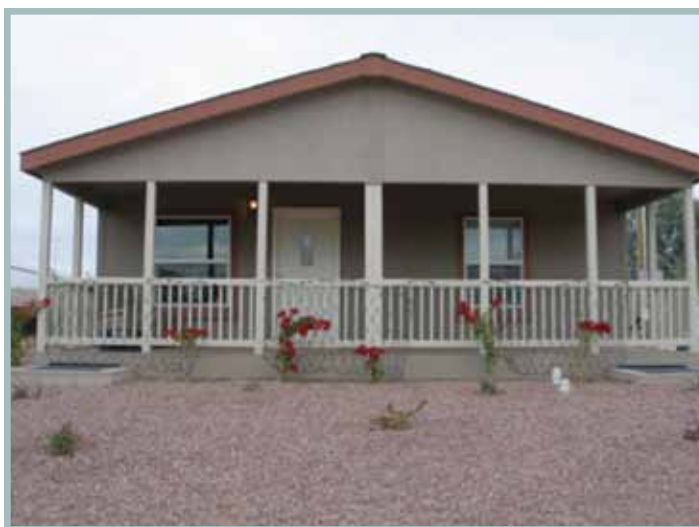
Primavera replaced this deteriorated house on West 38th Street with a new, attractive energy-efficient unit.
